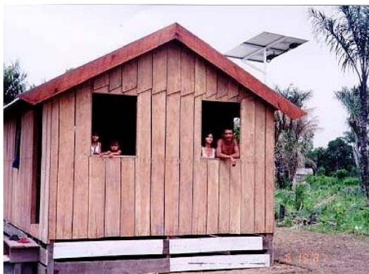
Fig.3: PV Solar Home System installed at a residence in one of the communities.
